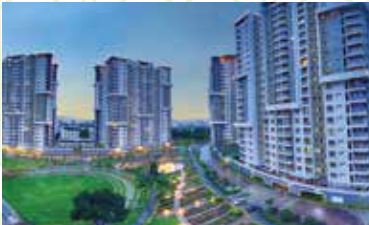
GREENAGE Hosur Main Road, Bengaluru
