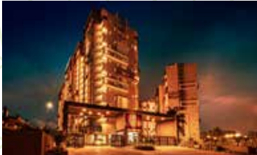
EAST CREST Near Budigere Cross, Bengaluru
